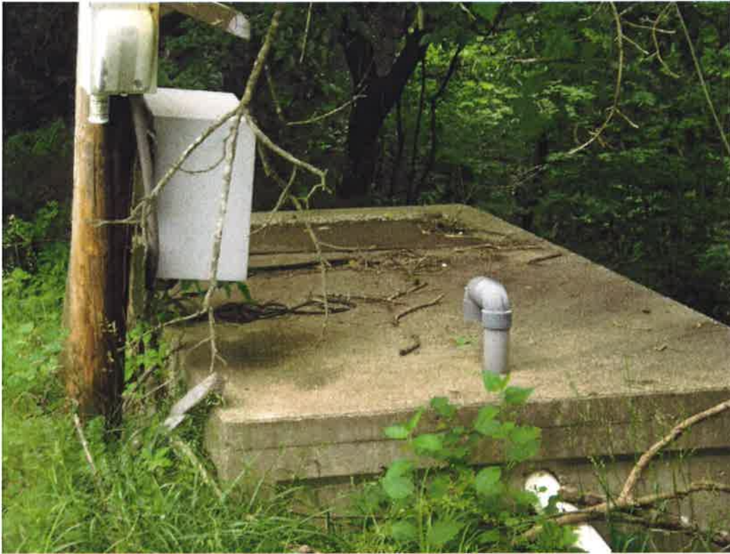
Existing Lift Station at Pool Area
